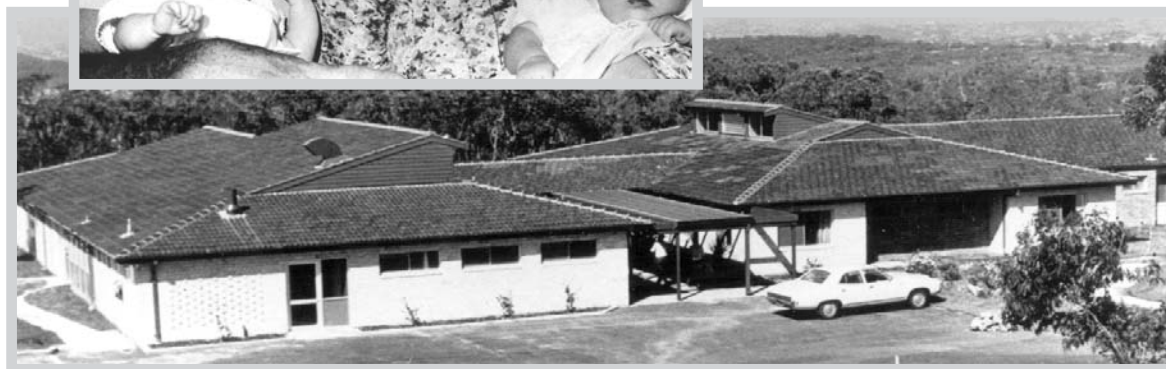
The completed hostel is surrounded by two miles of virgin bush and has a commanding view of the City.
